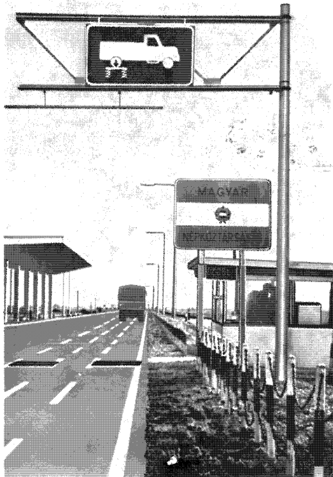
Fig. 1. Axle and wheel load checking scale installed at a boundary passage station
