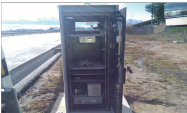
Fig. 9 Standard cabin for the assessment of speedometers
