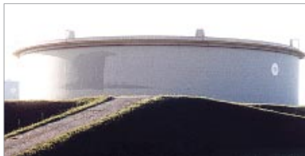
Fig. 5 View of the large storage tank used as test measure
